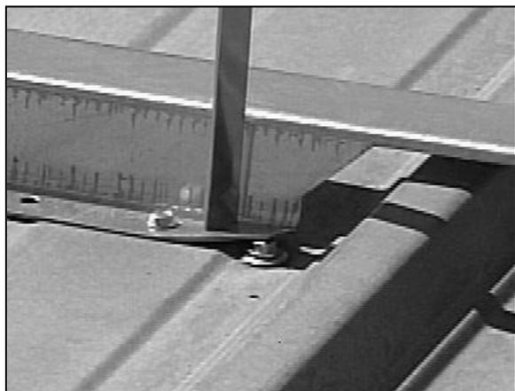
*(Typical “R” Panel installation showing the bending of the bottom flange caused by the existing fastener is normal.)*
