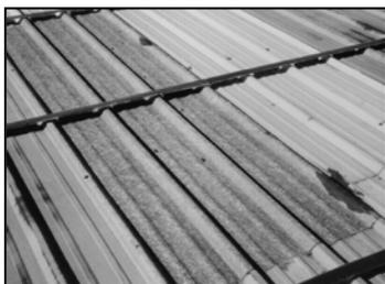
If skylights are to be installed where interior condensation could be an issue, it is desirable to replace the old skylight with a new one and install another new skylight above it to minimize any condensation issues in this area. Consult your local moisture control professional.
