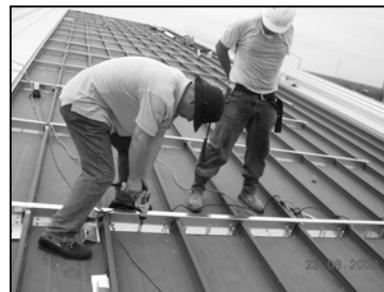
fasteners in addition to the clip fasteners or back lap the HUGGERS one full corrugation to produce a double thickness and continuity of the top flange across the lap.
