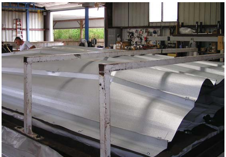
Testing after panel failure.
