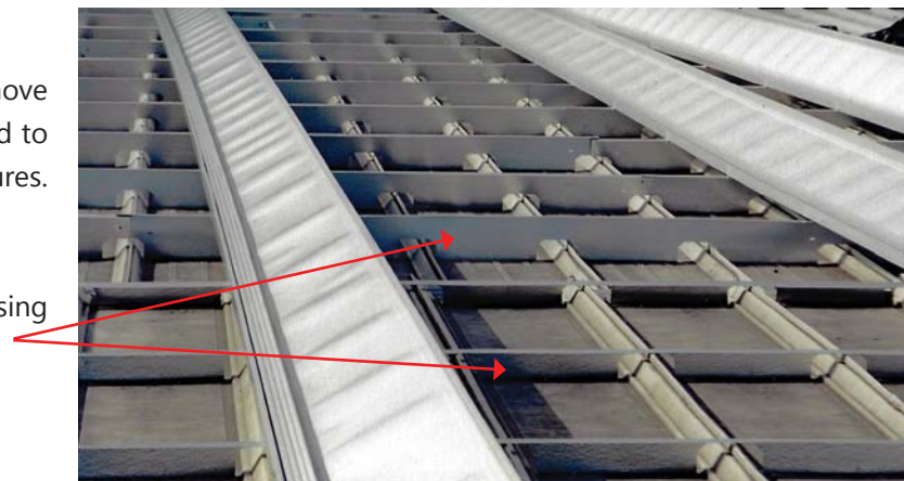
Using any 2 different height Roof Huggers to remove a roof step.
