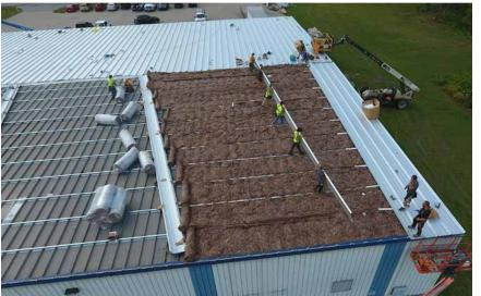
are not working over open framing which requires more equipment while exposing them to increased fall hazard, they are working on top of the existing roof. This makes stacking of material, equipment, tools, etc. much faster and easier.
