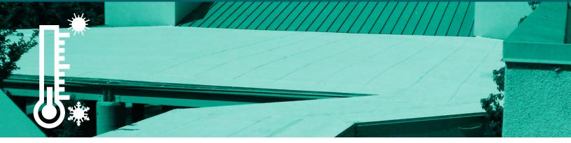
THERMastic built-up roofing systems and hot POWERply roofing systems are exceptionally durable and watertight. THERMastic systems are made of multiple plies adhered with high quality, enhanced THERMastic hot-melt adhesive that is far superior to regular mopping asphalt for elongation, low temperature flexibility and adhesion. Hot POWERply systems consist of two or more modified bitumen plies adhered in THERMastic adhesive.
