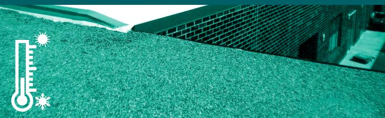
The PowerFAST Modified Bitumen (MB) System consists of a POWERply cap sheet membrane adhered to a high-performance POWERply anchor membrane, mechanically attached directly to the deck This configuration enables the PowerFAST roof system to become watertight quickly as well as providing wind uplift resistance that is superior to many fully adhered MB systems.
