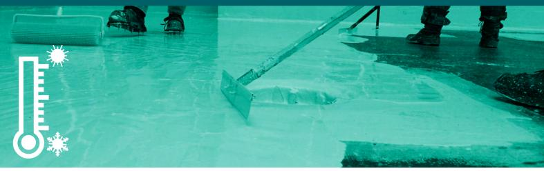
The two coat AlphaGuard PUMA Liquid Applied Roofing System can restore a variety of roof types and works just as well as a new or replacement roof. AlphaGuard PUMA is the perfect choice when you must work in temperatures as low as -20°F (-28°C). It can deliver waterproofing in as little as 30 minutes, accepts foot traffic after only one to two hours, and is fully cured in two days. Tremendous benefits at any time but especially in the bitter cold.
