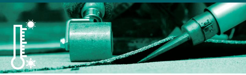
Our heat welded modified bitumen system, part of the POWERply\* line, consists of two or three MB sheets installed on the roof without adhesives. A propane torch or hot air welding equipment is used to weld the base membrane to a coverboard or a cap sheet to a base membrane. The remainder of the roofing system, including insulation and coverboard, can be adhered with hot asphalt, low rise foam insulation adhesive or mechanical fasteners.
