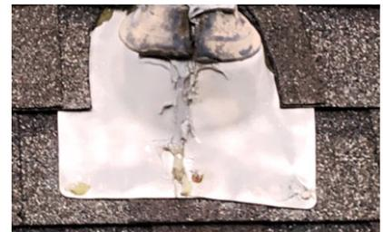
*Damaged or aged roof jacks may allow water leaks in your roof.*
