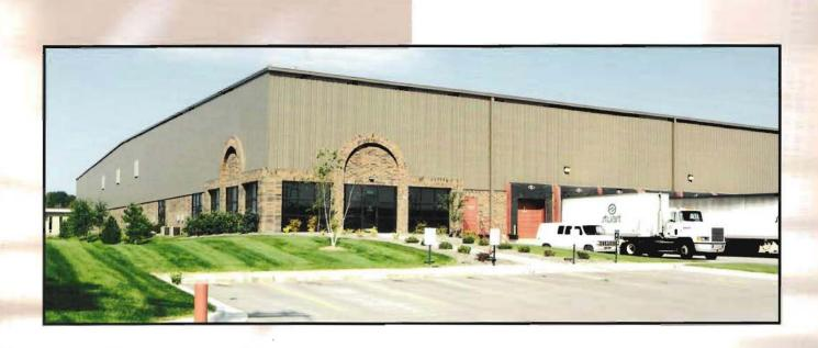
Metal buildings also minimize the use of columns ... while still meeting the needs for rack storage, conveyor belts, crane systems, mezzanines for office areas or additional storage. And when large expanses are needed, long-bay systems can be designed with columns spaced far apart.
