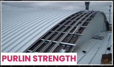
**Roof Hugger Sub-Purlins Have The Ability** To Add Strength To The Existing Purlins. This Is Important Because Most Retrofit Systems Just Add Weight.
