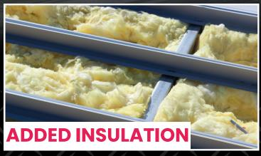
When you install Roof Huggers, the air space between the existing old roof and the bottom side of the new roof is well suited to install insulation for increasing the building's thermal resistance.
